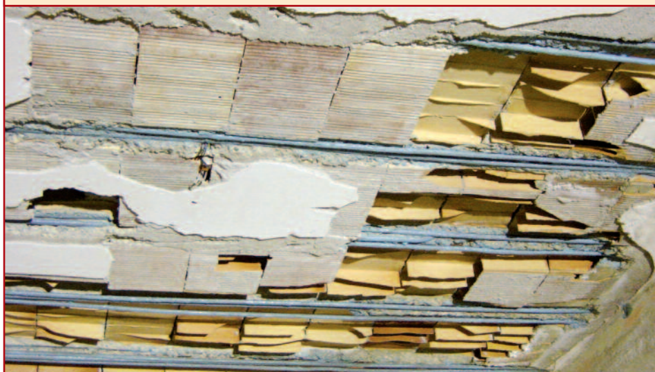
[FIG. 4] - Trattamento armature / Rods Treatment
